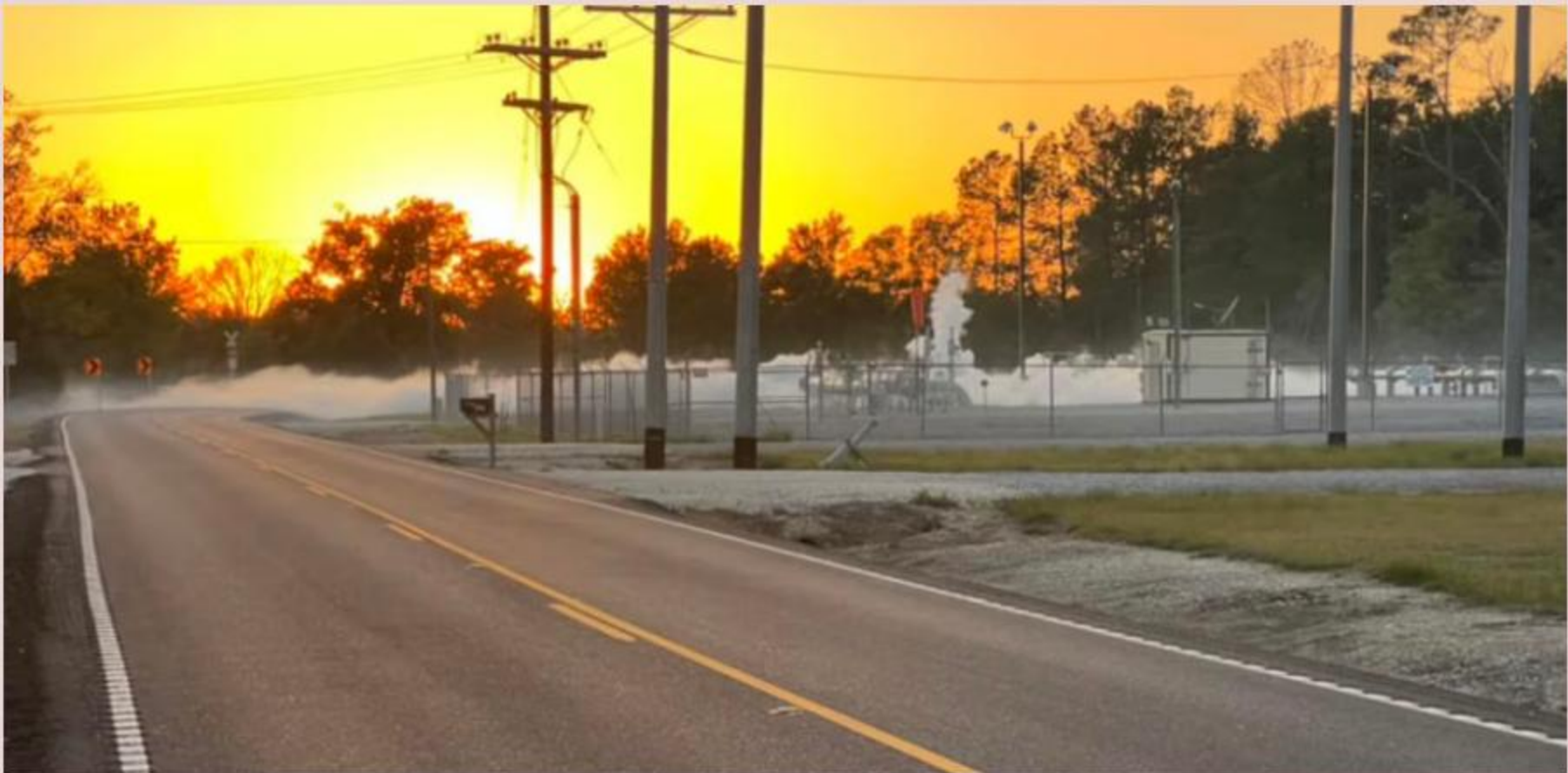
Denbury CO2 pipeline leak near Sulphur, La. on April 3. (Image: Calcasieu Parish Police Jury )
